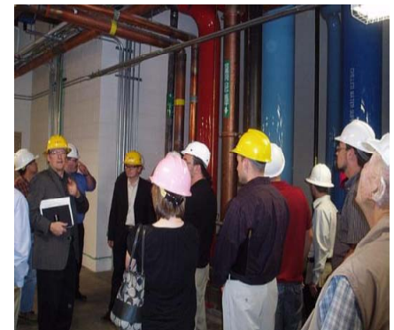
February Central Plant Tour at Phoenix Children's Hospital
